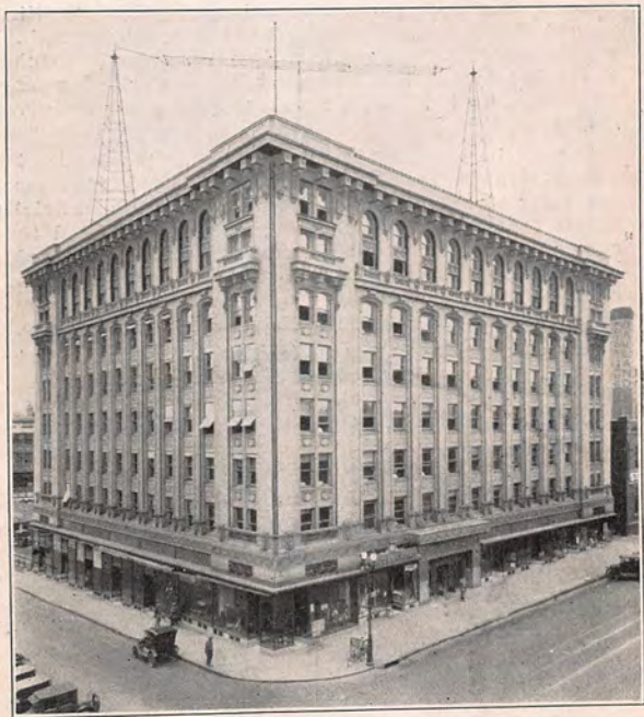
GRAIN EXCHANGE BUILDING
