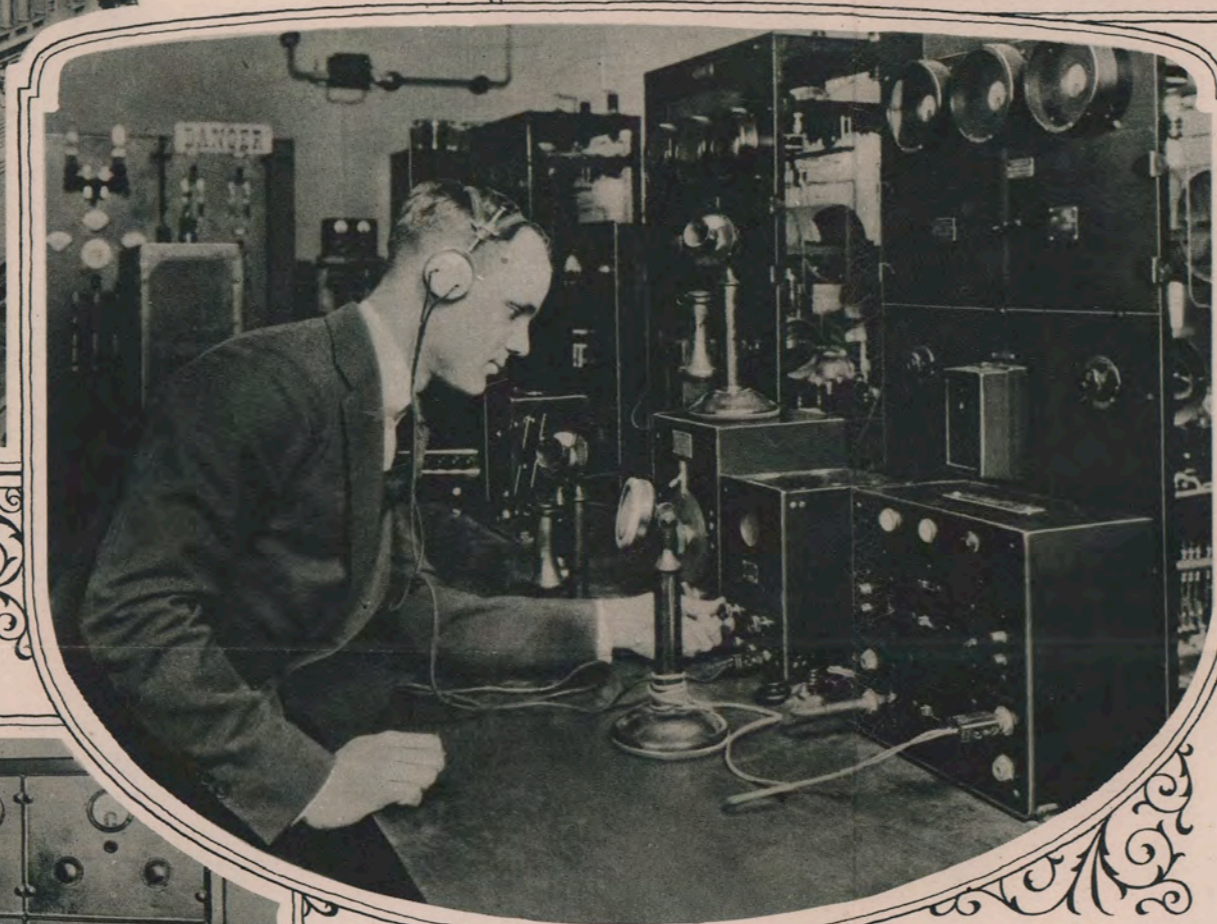
A View of the Station Room on the Roof
