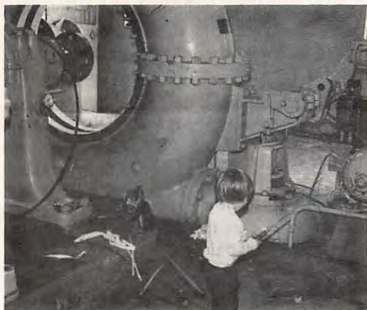
HCJB generator under repair
