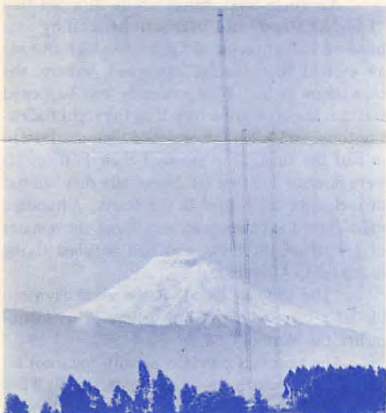
Main tower of Steerable Antenna with Cotopaxi in background
