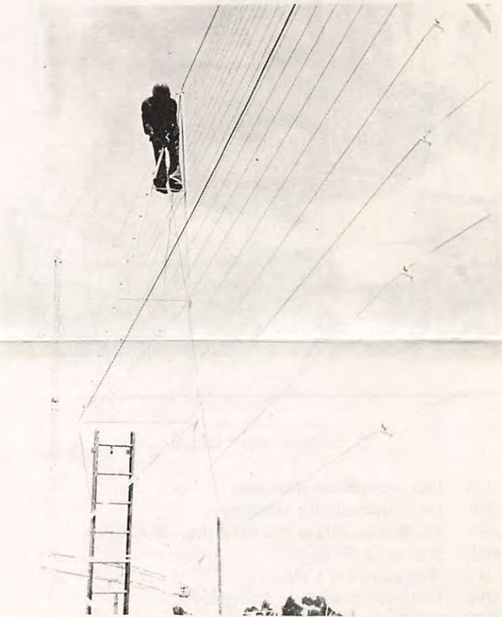
The stringing of wires for the corner reflector in which the bi-conical dipole is located.
