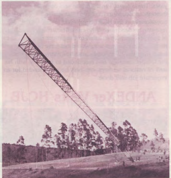
Tower raising in July for HCJB's new North-South America antenna
