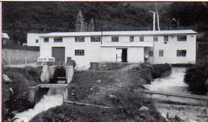
HCJB's hydroelectric plant
