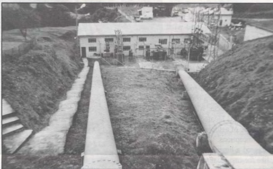
Penstock leading into generator building in Papallacta.
