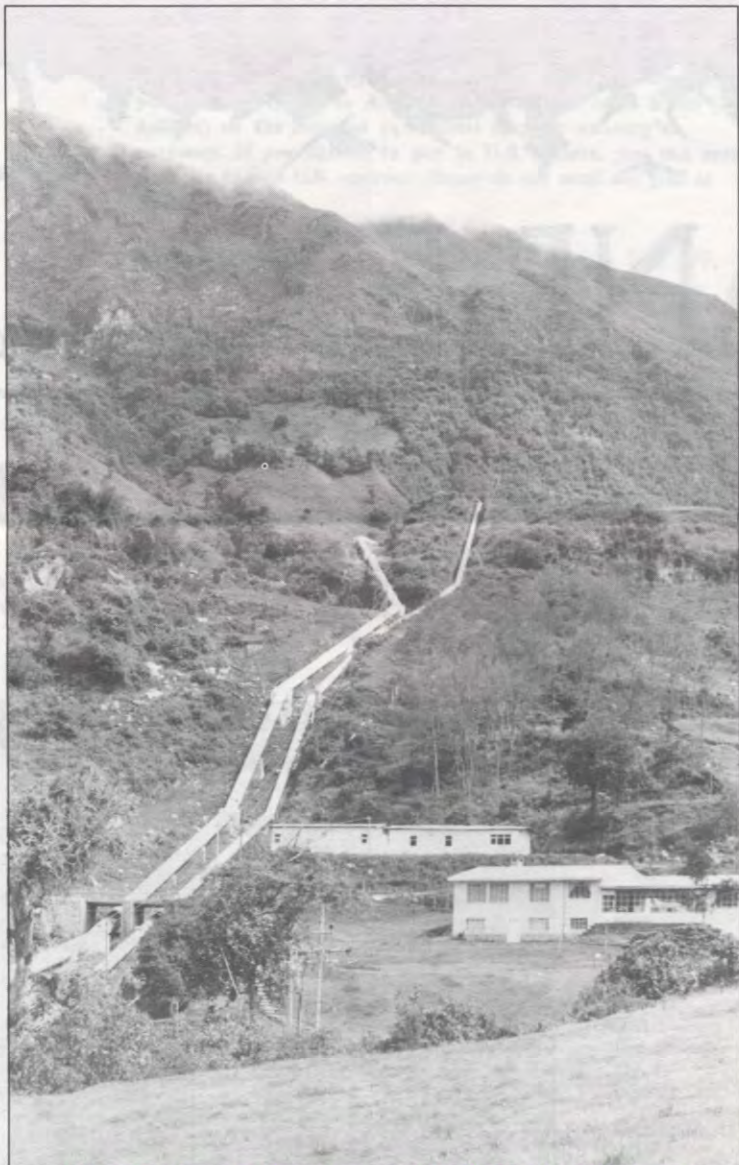
1,400-foot-long (430-meter) and 1,903-foot (580-meter) penstock - Papallacta
