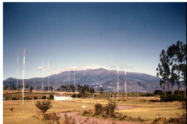
Huge curtain antennas at HCJB's Pifo transmitter site high in the Andes mountains sent Christian programming around the world via shortwave.
