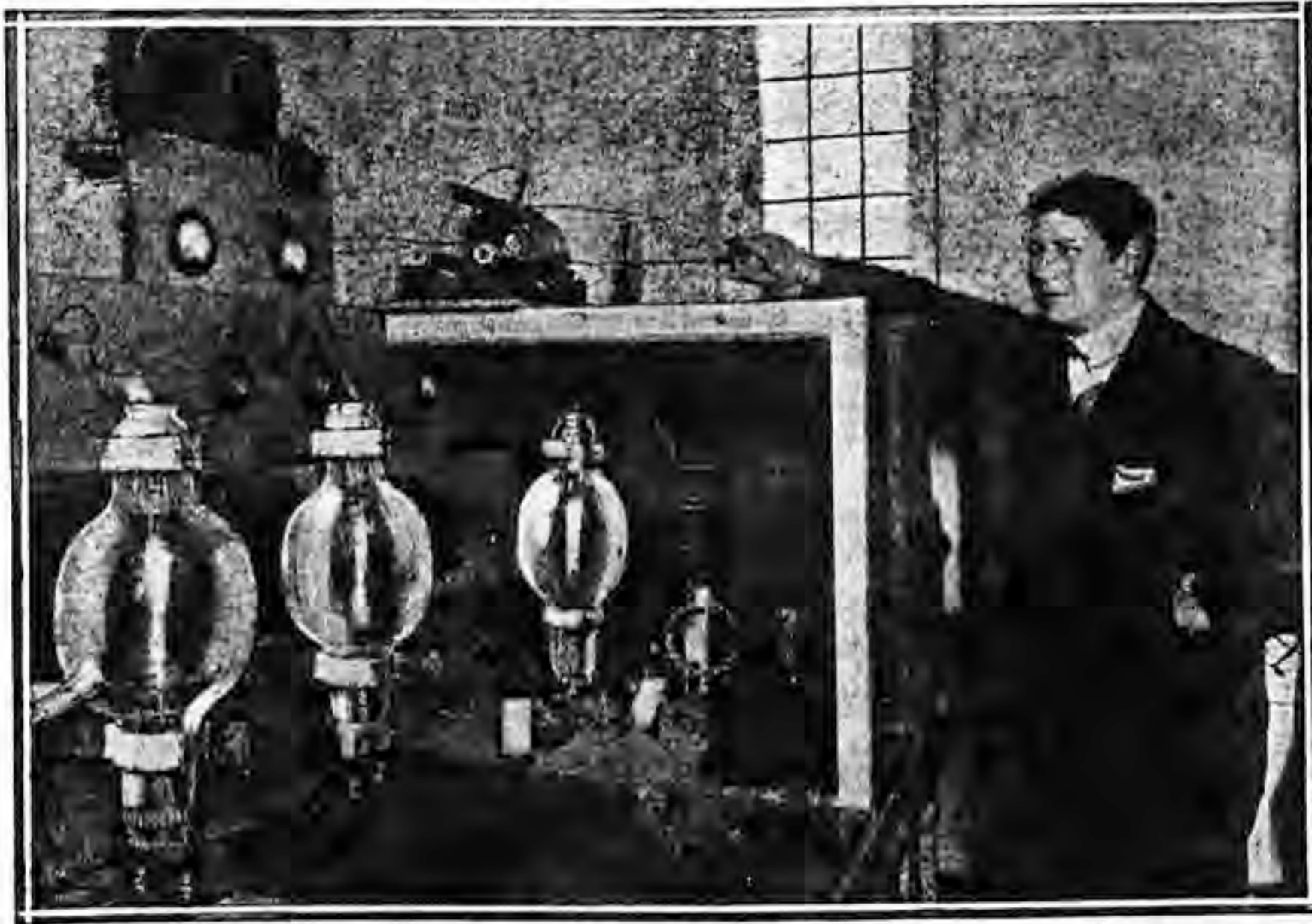
The transmitter of G2NM, located at Coombe Dingle, Caterham, Surrey, England, a few miles to the south and west of London. This 1,200-watt station has been heard in all parts of the world. Its call was familiar to all amateurs long before Mr. Marcuse undertook short-wave broadcasting for the benefit of listeners throughout the British Empire—and incidentally others.
