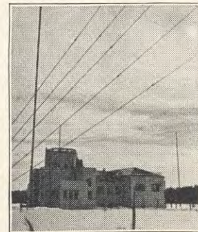
COMINTERN BROADCASTING STATION
