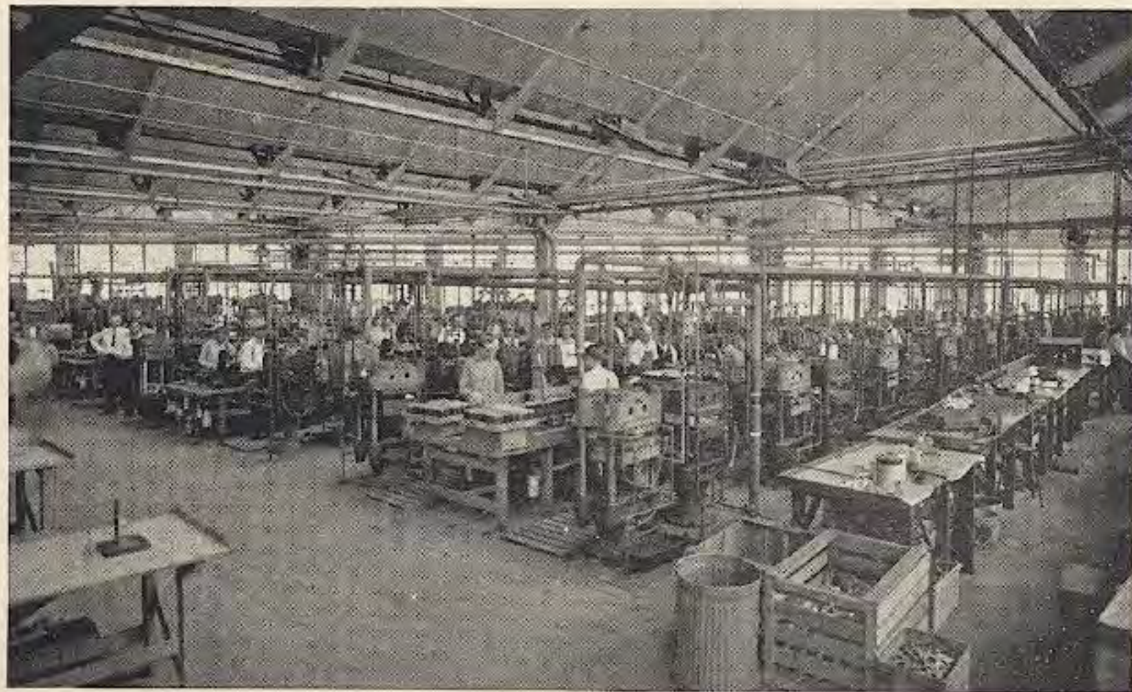
Bakelite moulding department—the largest privately owned Bakelite moulding plant in the world.
