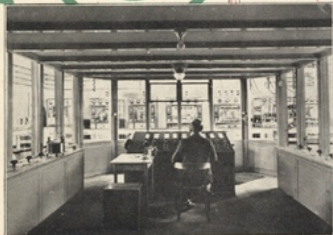
A VIEW IN THE CONTROL-ROOM OF THE PHOHI TRANSMITTER
