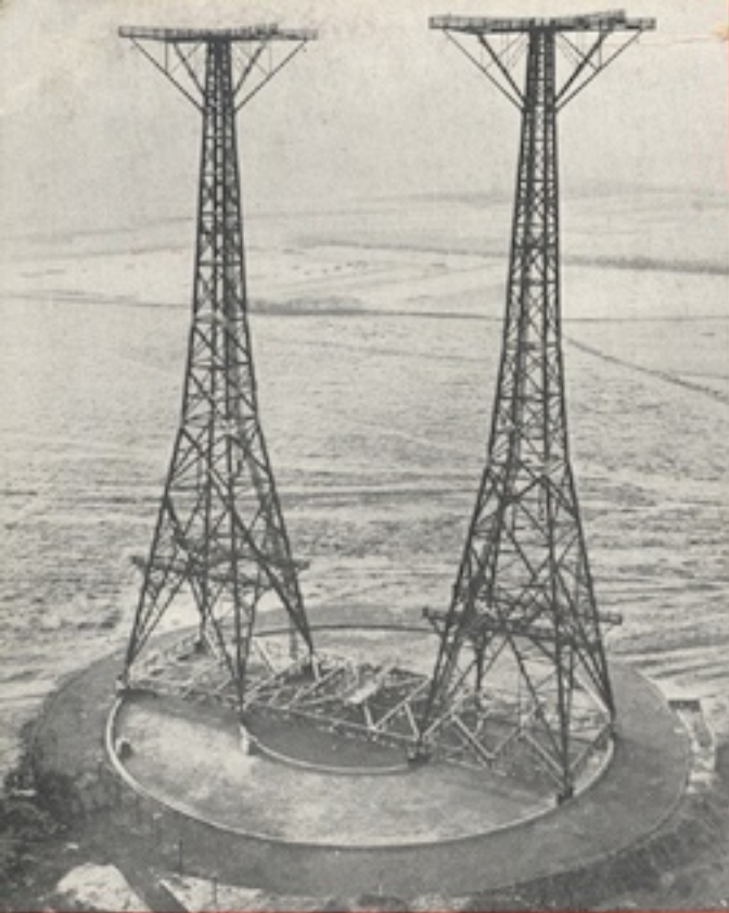
P.C.J.'s aerial masts on wheels, which can be directed to every part of the world.
