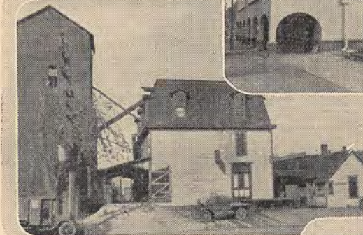
The mill property which we recently got and will probably remodel as soon as possible to make it fit our needs.
