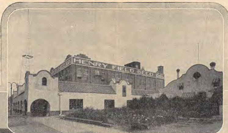
This is Seed House No. 1 and the Studio and shows the New Arcade store building connecting them.
