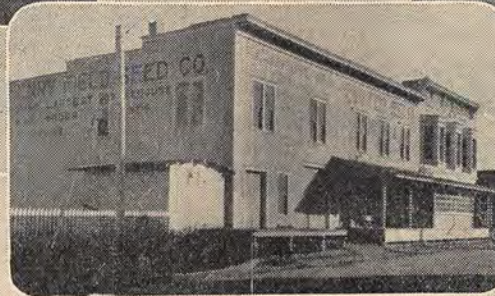
Above — No. 4 Building where you'll find the Fencing, Roofing and other things. Right — No. 5 Building where the Garden seeds, Bulbs and Merchandise are shipped from.
