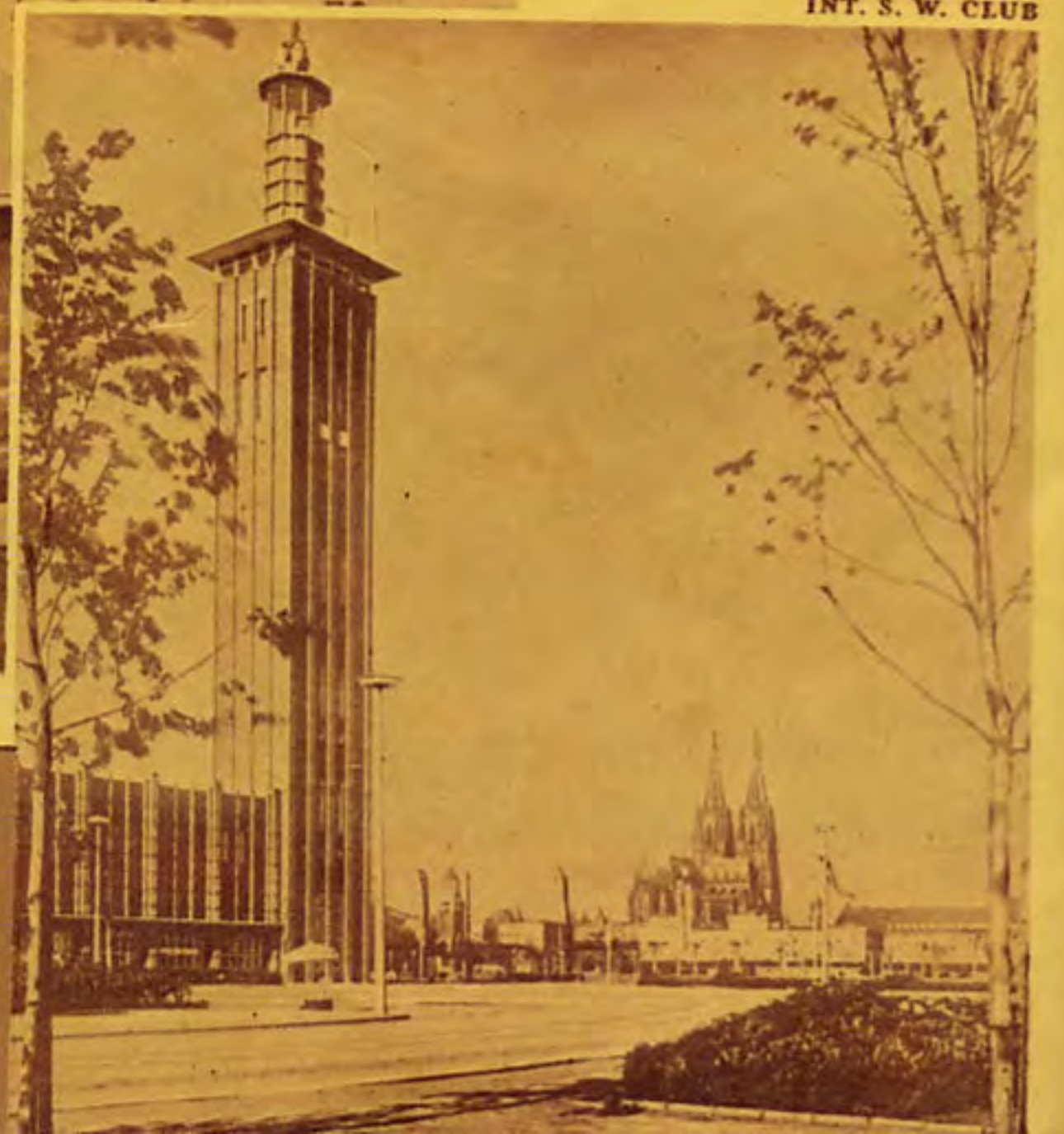
Even radio stations have gone modernistic in Nazi Germany. At the right is seen the studios and transmitting tower of a recently completed station in Cologne. The famous Cologne cathedral is in the background.
