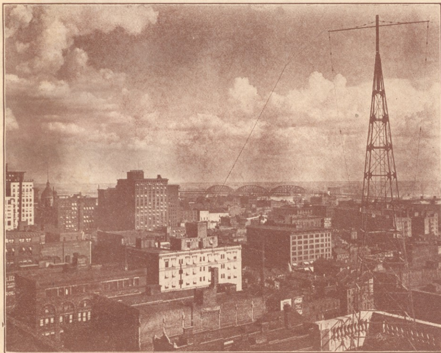
How the radio towers of K S D, on the roof of the Post-Dispatch Building, dominate the skyline of St. Louis. These towers are 100 feet high (to tip of wooden mast) and 14 feet square at the base. The four legs go through the roof of the building to be anchored upon the steel framework of the structure itself. A powerful winch at the base of each tower makes it possible to stretch the phosphor-bronze aerial as tight as a violin string.
