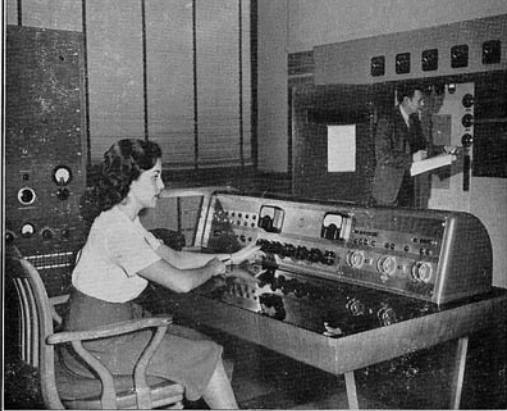
(Above) Some of the Aerials. (Below) One of the Control Panels.
