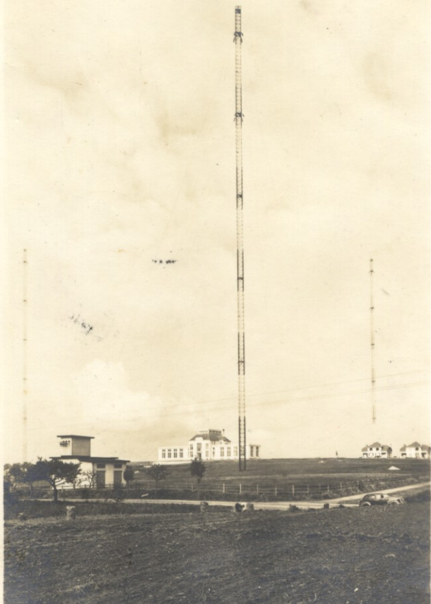
TRANSMITTING STATION RADIO LUXEMBOURG.
