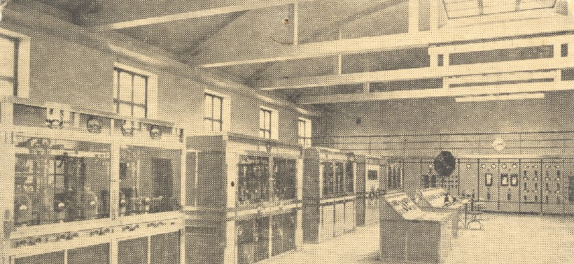
Lehti Bc Station 160 Kc 250 Kw. Made in Marconi England 1932. Director O H 3 P P. Second Bc Stu 100 Kw 15190 Kc Made in Finland 1948.
