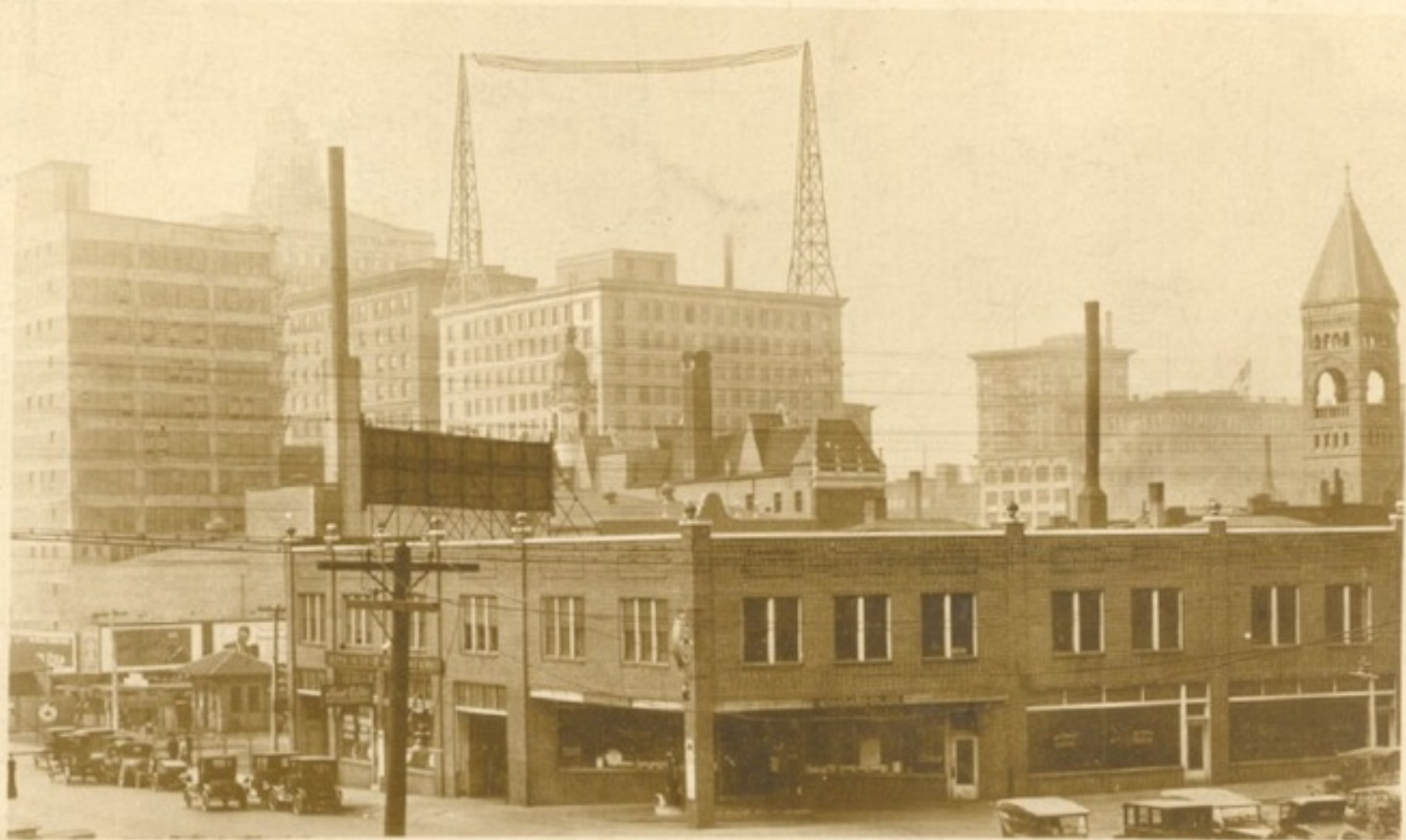
RADIO BROADCASTING TOWERS, BANKERS LIFE COMPANY, DES MOINES, IOWA
