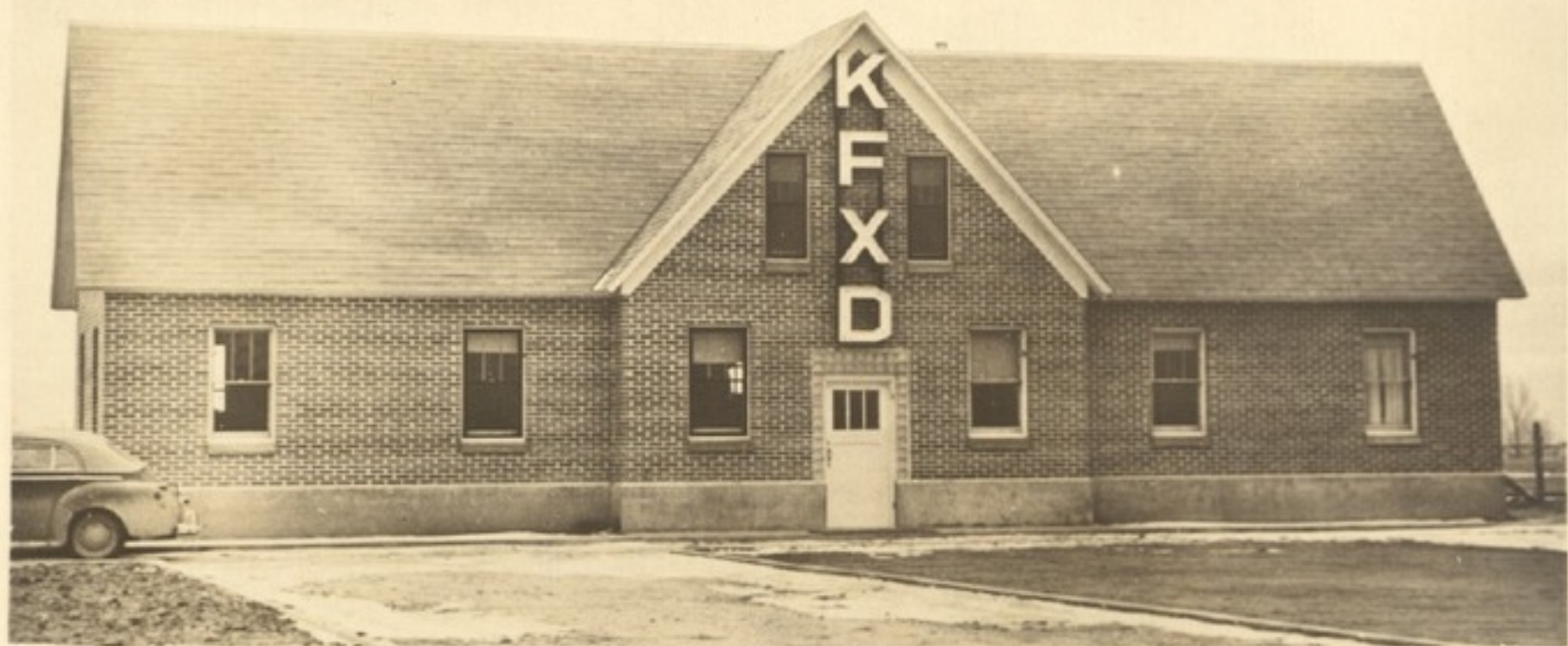
The New KFXD transmitter building, housing the new 1000 watt AM transmitter and 2500 watt FM transmitter
