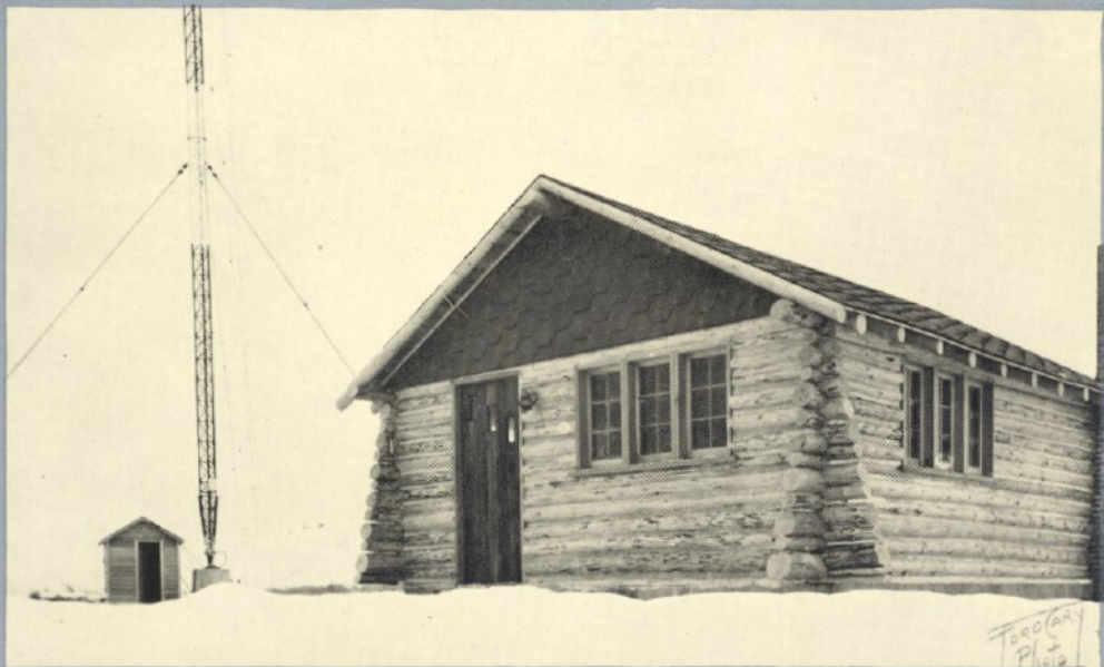
EXTERIOR OF TRANSMITTER BUILDING SHOWING BASE OF 307 FT. TOWER. WTCM, TRAVERSE CITY, MICH.
