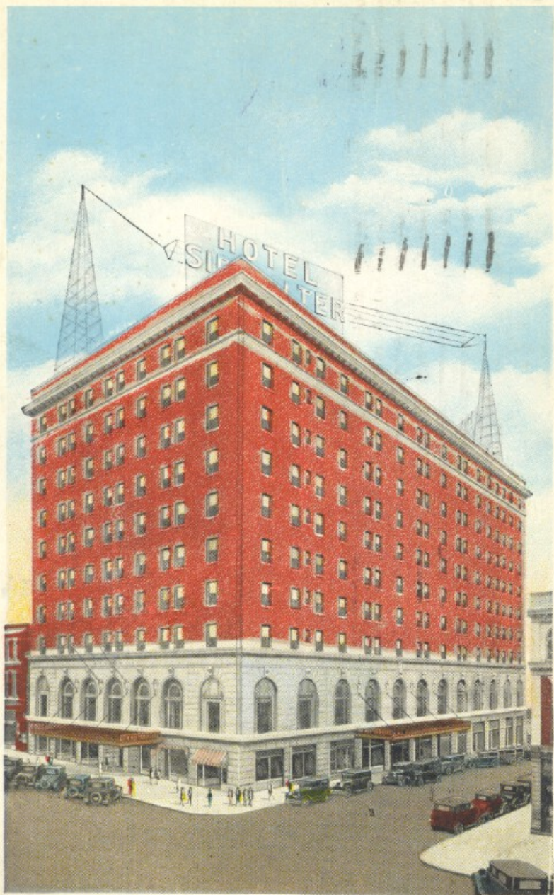
SIR WALTER HOTEL AND ANTENNA OF RADIO STATION W. P. T. F., RALEIGH, N. C.
