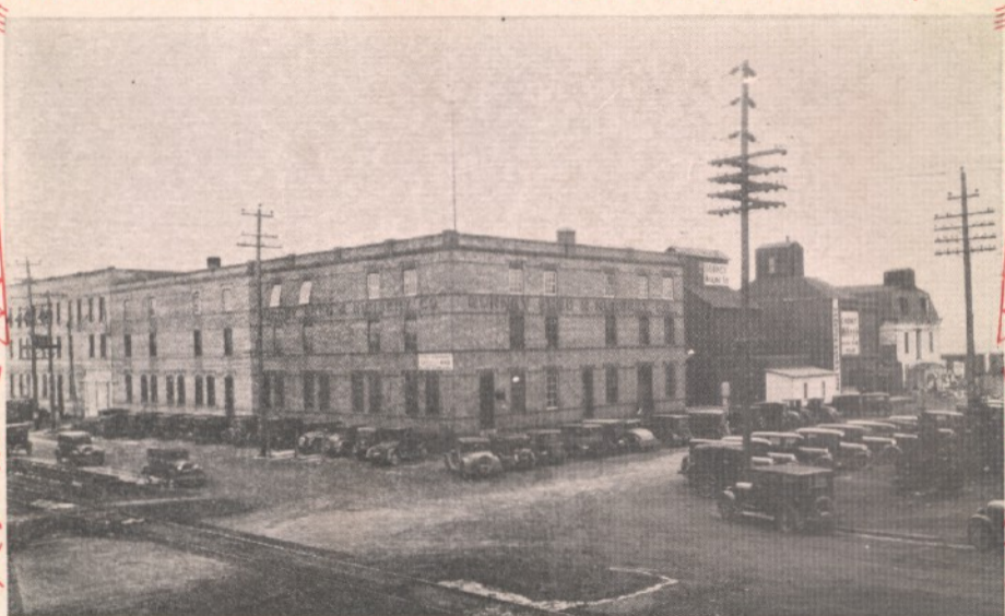
A good week-day picture of our Main Building. On Sundays thousands of cars park as near to us as possible.
