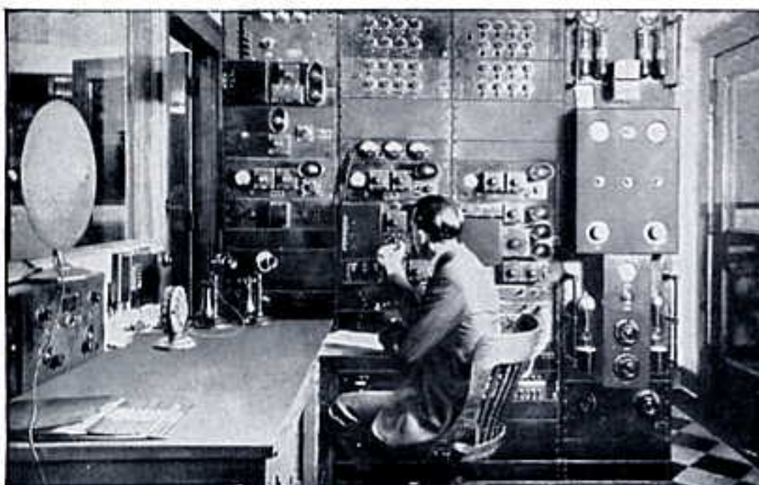
WOC Control Room
