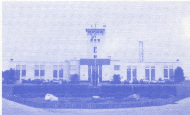
VOA BETHANY RELAY STATION MASON, OHIO
