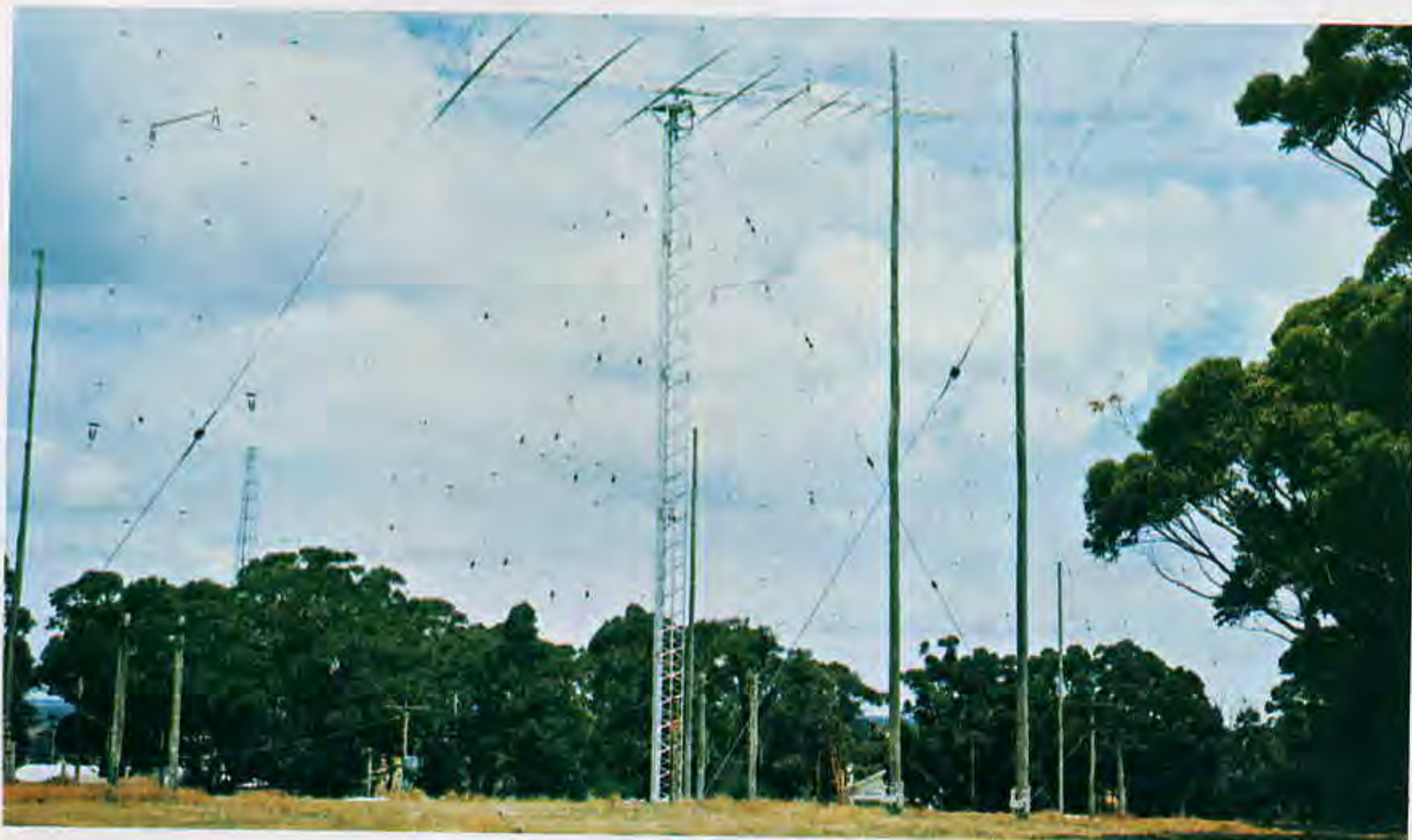
Transmitters at Lyndhurst
