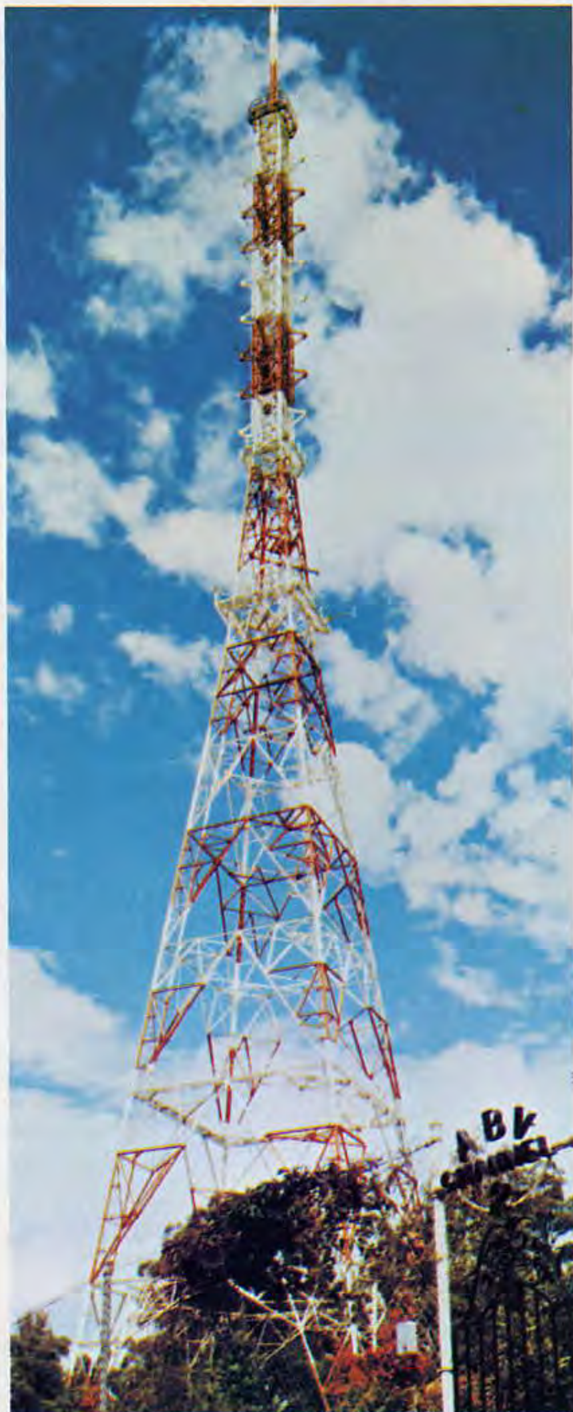
ABV2 transmitter station at Mount Dandenong
