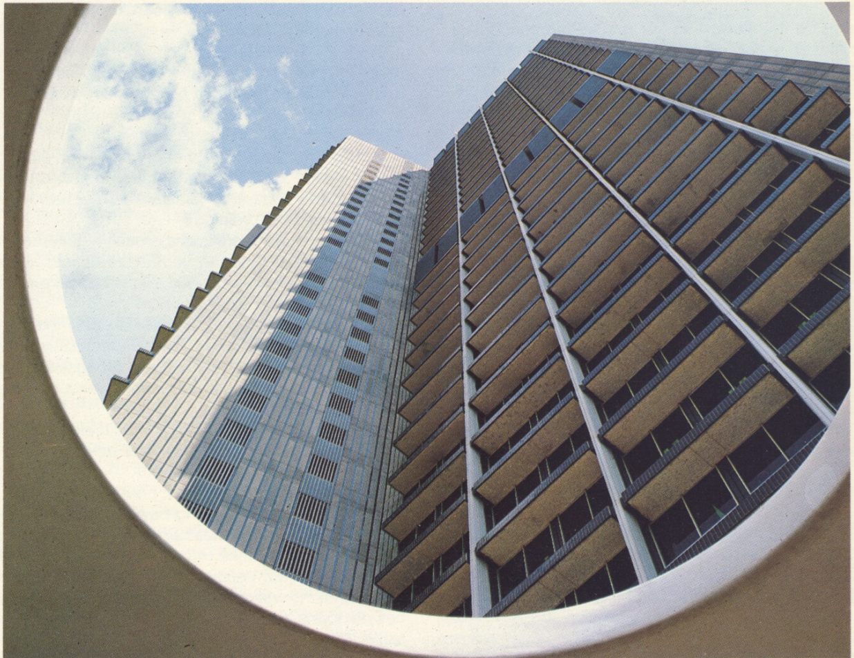
The tower block from the piazza level at Broadcasting Centre.
