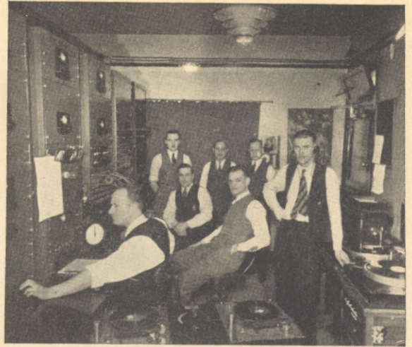
CFRB MAIN CONTROL ROOM
