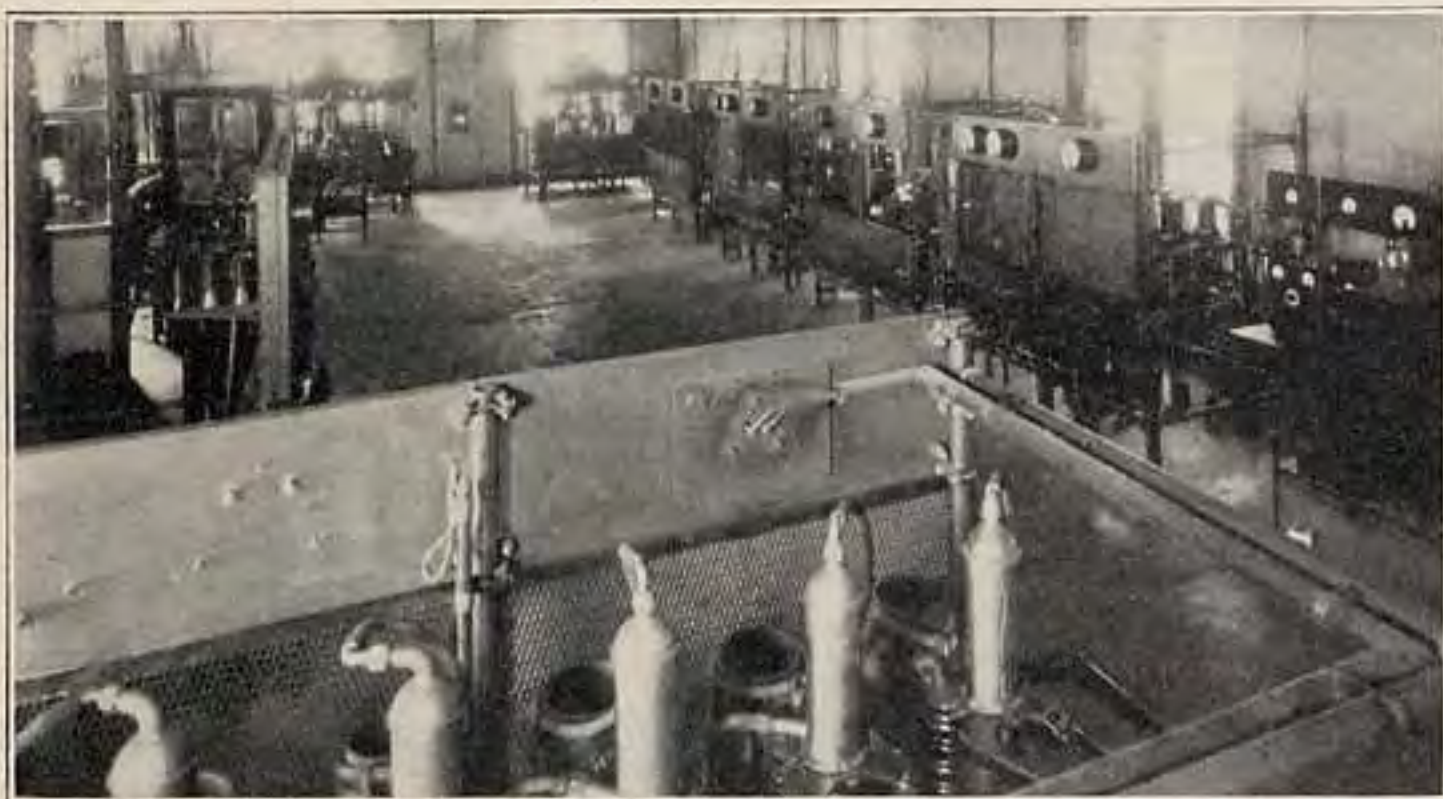
Interior view of transmitting station of Westinghouse KDKA, showing amplifiers, modulators, and oscillator panels. Water-cooled tubes of a short-wave transmitter appear in left foreground.
