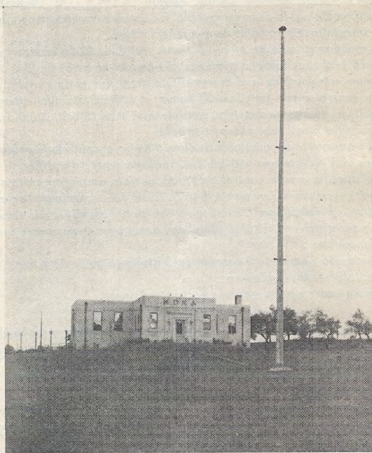
Fig. 1—Front view of Westinghouse radio station at Saxonburg, Pa.
