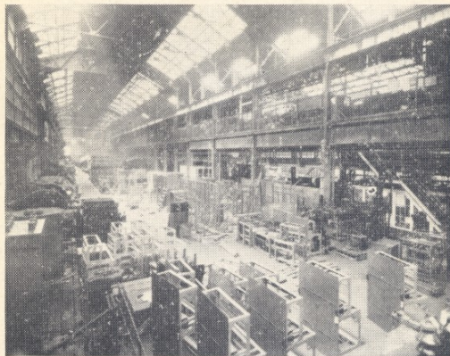
Interior view of Main Works, Westinghouse Electric & Mfg. Co., East Pittsburgh, where Truck Type Switchboards are assembled.
