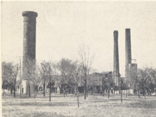
Hastings Municipal Electric Light and Power Plant, which furnishes power for KFKX
