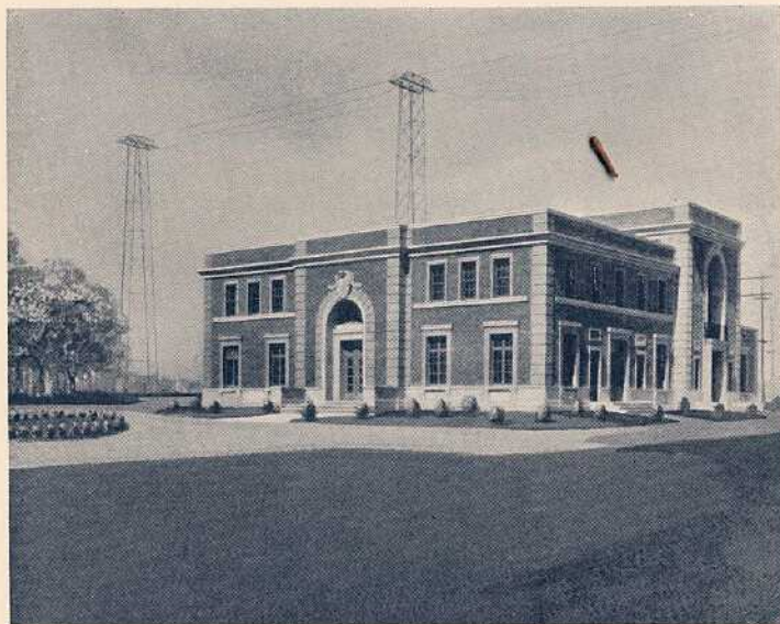
Main Building at Lawrenceville, housing two of the transmitters
