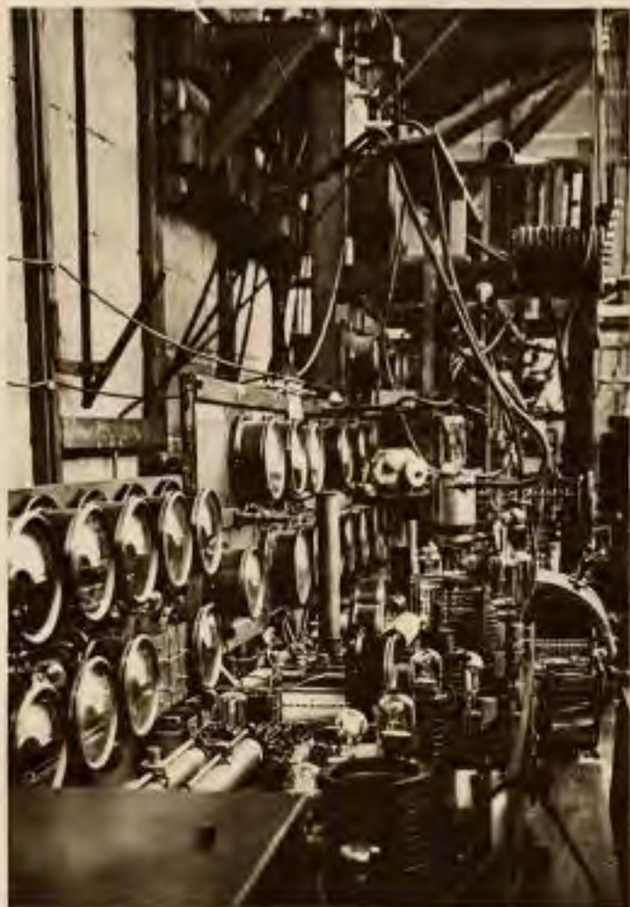
Crystal oscillator and multiplying stages
