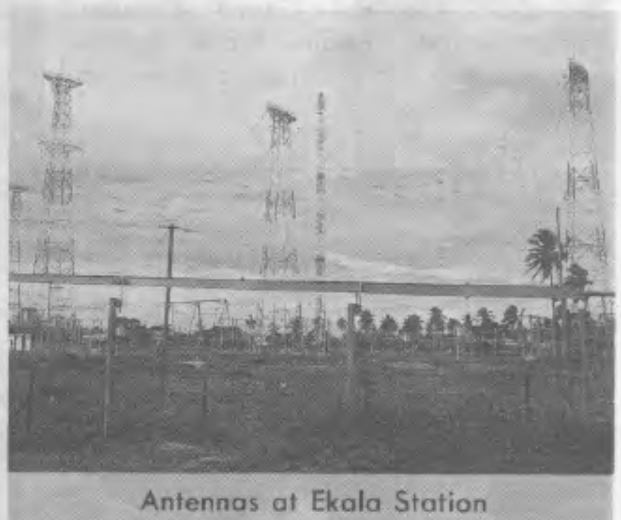
Antennas at Ekala Station
