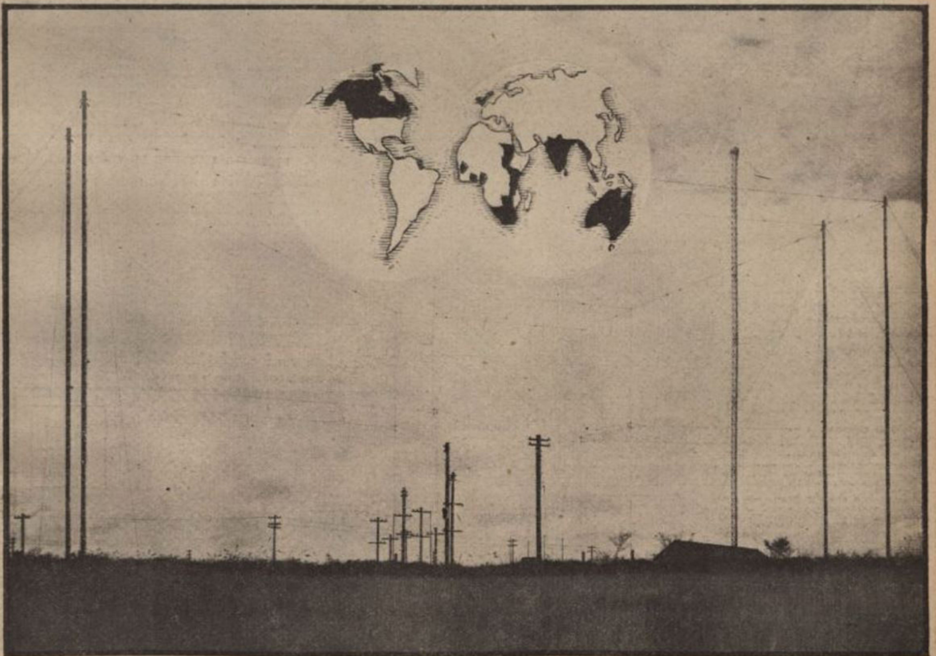
On December 19, the new Empire Broadcasting Station at Daventry opens a regular service of special programmes for the Dominions and Colonies. Our photograph shows the aerials for the Australasian Zone.
