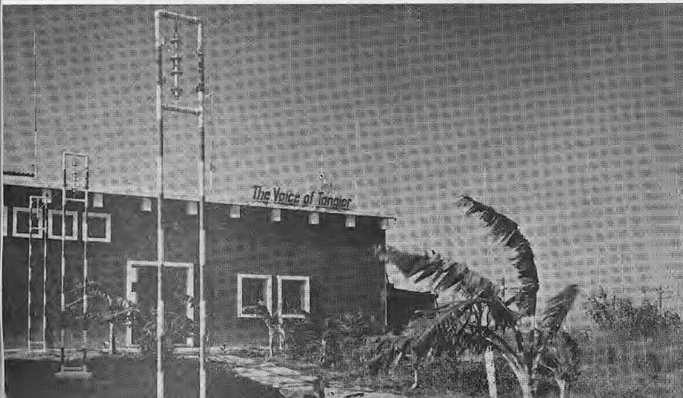
Transmitter Building in Tangier
