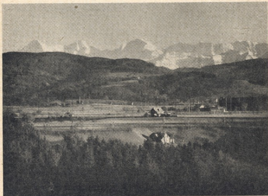
General view of S.B.C. transmitting station at Schwarzenburg, Berne
