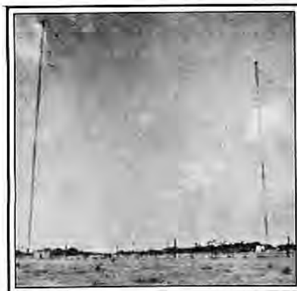
The antenna system at Radio Americas.
