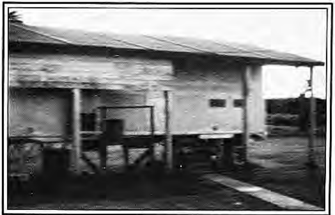
Another view of one of the transmitter vans.
