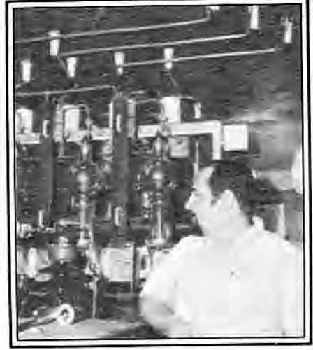
The RA transmitter had six gigantic tubes in the final amplifier stage. The signals head for the antenna via heavy cables overhead.
