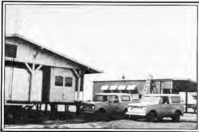
RA's transmitters were all in vans parked under a common roof. The generator building is at the rear.
