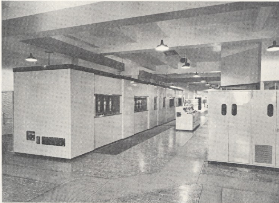
Figure 3 — Part of transmitter room of the VOA Philippines Relay Station showing Machlett ML-5682's in Continental 1 Mw medium-wave transmitter which broadcasts to Asia on 1140 kc.
