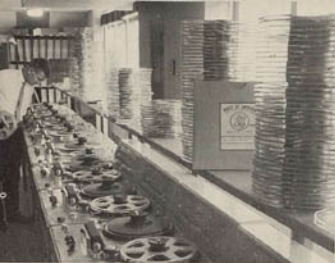
These machines are used to make multiple copies of Voice programs at high speed, facilitating shipment of recordings for placement on foreign radio stations.
