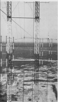
Antenna towers at Greenville.
