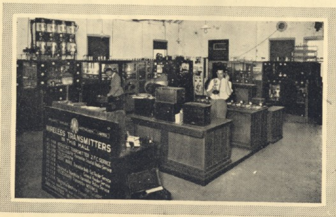
Section of Transmitting Room at A.W.A. Radio Centre, Pennant Hills, Sydney.
