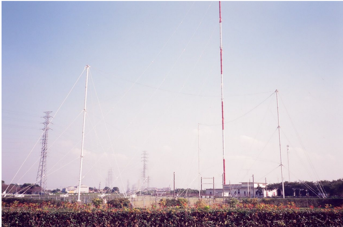
Shortwave antenna of NHK-Tokyo (Shobu-Kuki Radio Transmitting Station) in 1999
